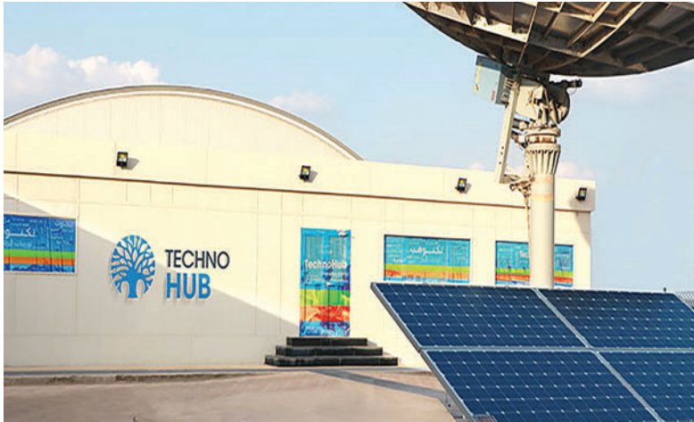
Gord Insitute research and development Technohub; Qatar Energy CEO and Qatar's State Minister at the inauguration event of the Al Kharsaah solar plant project
