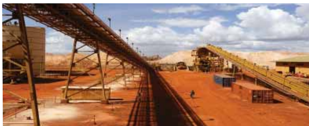
The processing plant at the Merian gold mine
