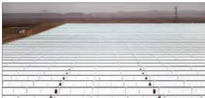
Morocco: The Ouarzazate solar power complex supported by the EIB
