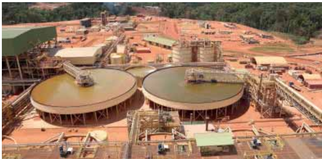
Newmont Mining processing facilities at Merian
