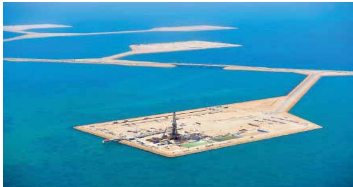
An island no longer Saudi Aramco's Manifa facility, Saudi Arabia
