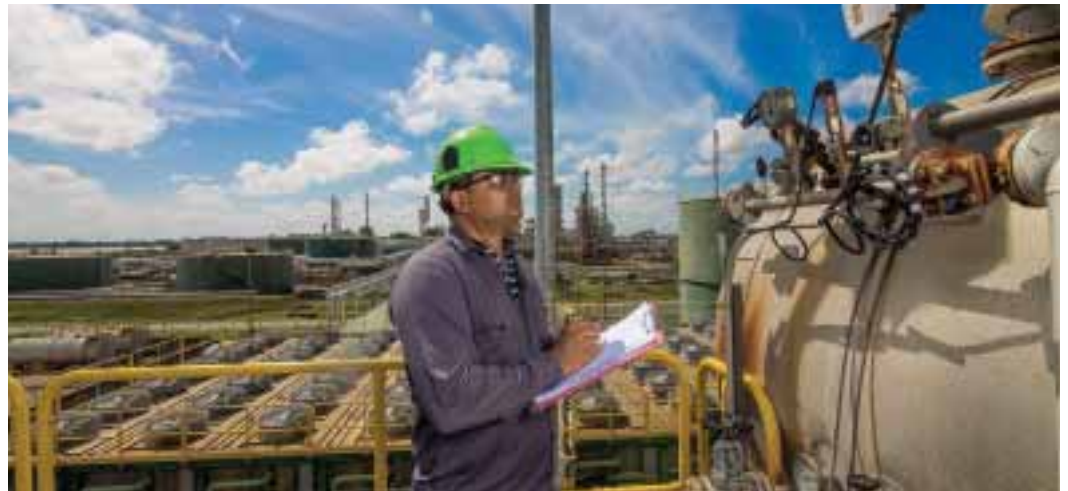
An employee of SPCS (Staatsolie thermal plant) at work with the refinery as background
