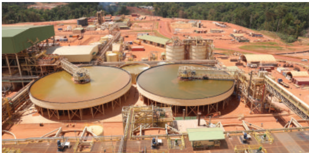
Newmont Mining processing facilities at Merian
