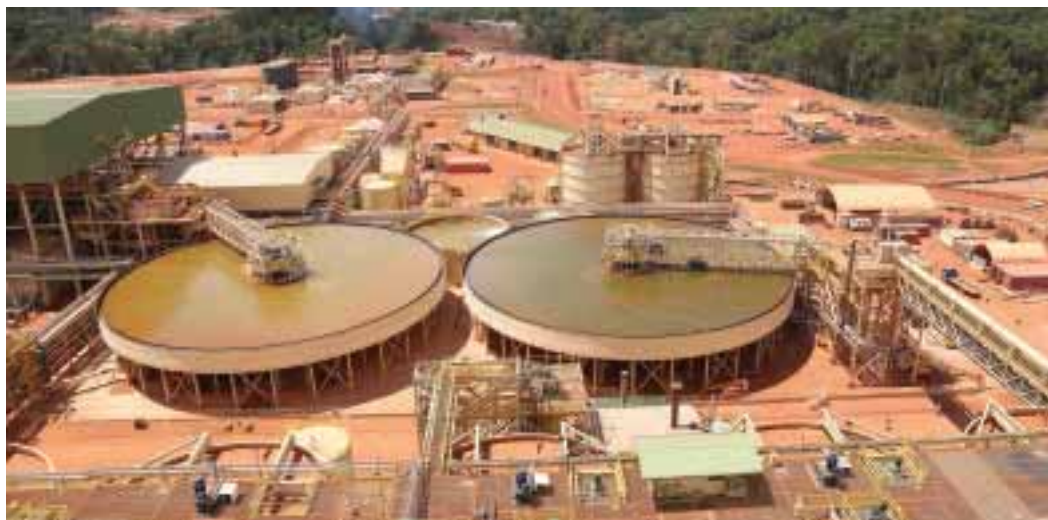
Newmont Mining processing facilities at Merian
