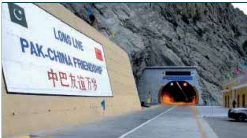
Karakoram Highway Tunnels
