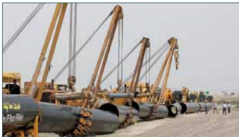
Sections of gas pipes are seen at the start of construction on a pipeline to transfer natural gas from Iran to Pakistan
