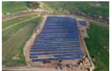
Solar power plant, Nisou
