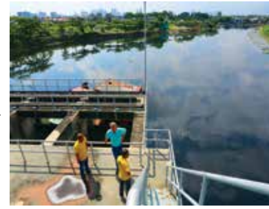
Metro Manila: pumping station to help reduce flooding
