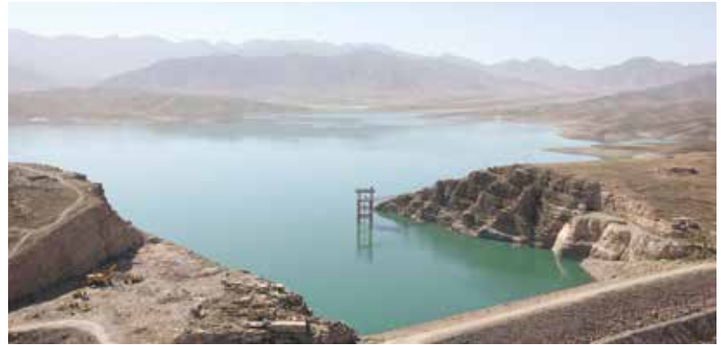
The Kajaki Hydroelectric dam project in Afghanistan, financed by the World Bank
